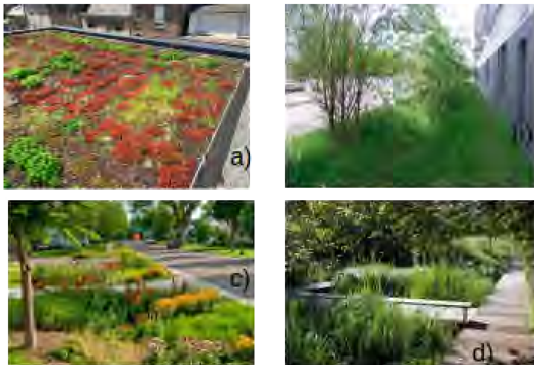
Figure 12 : Examples of NBS associated to stormwater management in urban areas - a) Green roof; b) Vegetated swale; c) Rain garden; d) Small bioretention basin
