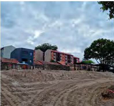
Figure 22: Removal and preservation of topsoil (20cm), and latter redistribution on graded areas, after earthworks.
