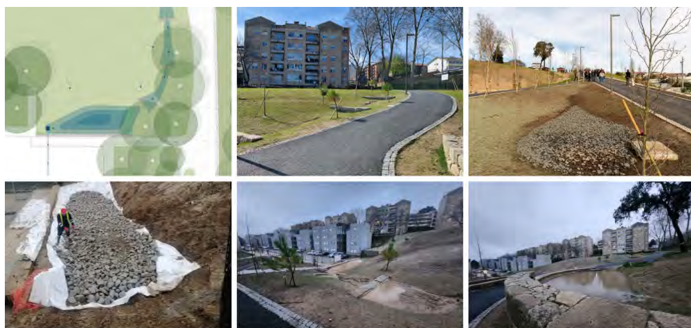
Figure 18: Stormwater management and infiltration NBS's (the system has already been tested during heavy rains, lower centre and right images).
